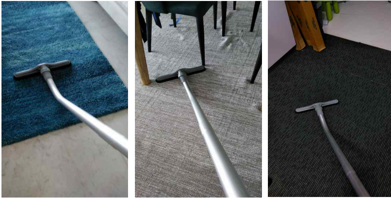
HEPA vacuuming before steam extraction/wet extraction
