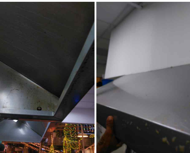
Degreasing the whole hood
