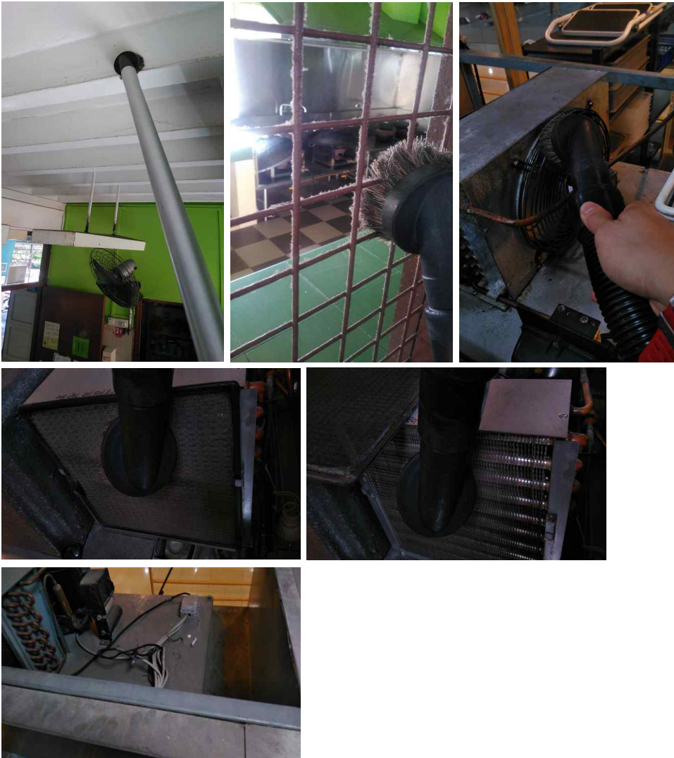
HEPA vacuuming for ceiling, fridge fan, grille, filter etc
