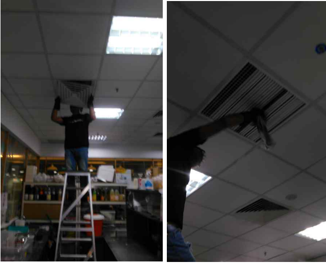
Take down all aircon grille and degrease front and back of the grille. Including the air return
