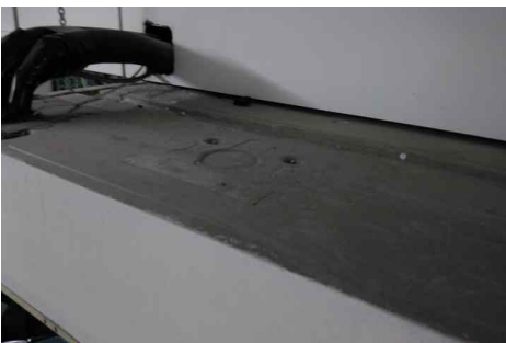
Dust build up on the top of aircon unit. Before and after. Video: https://youtu.be/ZbpFg5kYCTc
